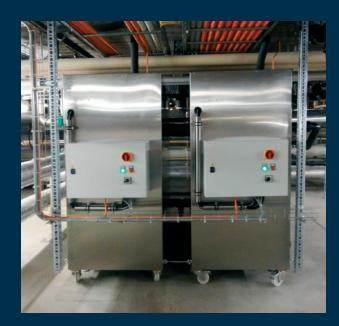
Several units can be connected to same system, if there is plenty of kettles to be cooled.
